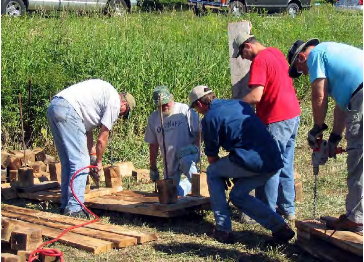
Lunker building site
